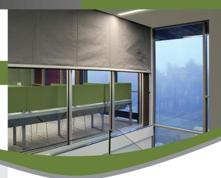
Codes and Standards. M2500 fulfills IBC requirements to provide an opening protective, where these assemblies are permitted as passive barriers used in conjunction with smoke control systems. This smoke-rated curtain system can serve as an opening protective for counter top, openings in corridor, and certain applications in atrium construction.
